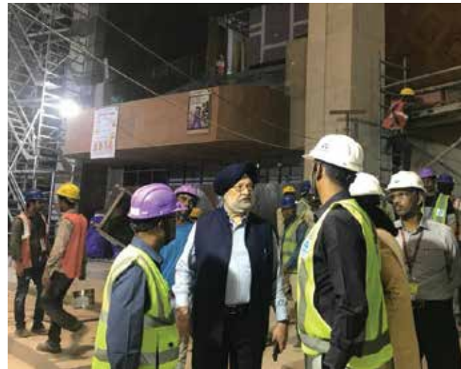
▲ Inspecting the construction of New Parliament building.
